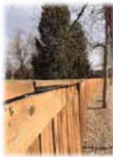
EXISTING FENCE (DAMAGED TOP RAIL)
